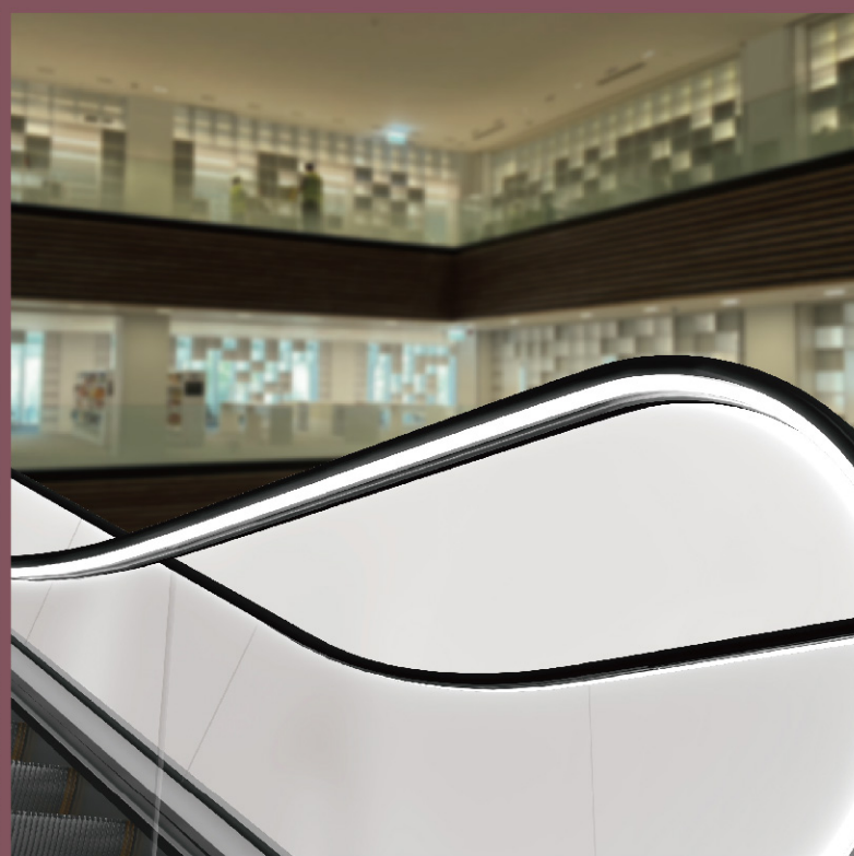
扶手照明 Handrail lighting
